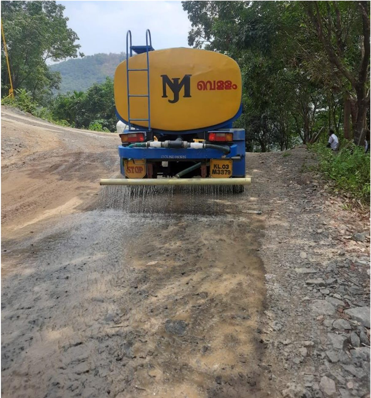
Plate G-4: Sprinklers and dust suppression methods adopted
